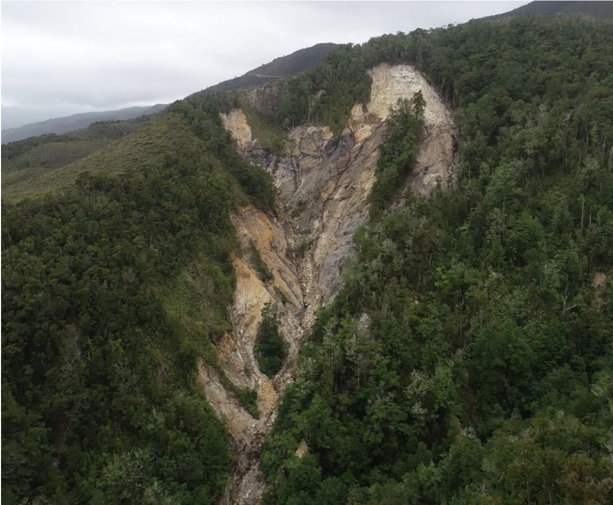
Slip in the upper catchment of Lake Stream
